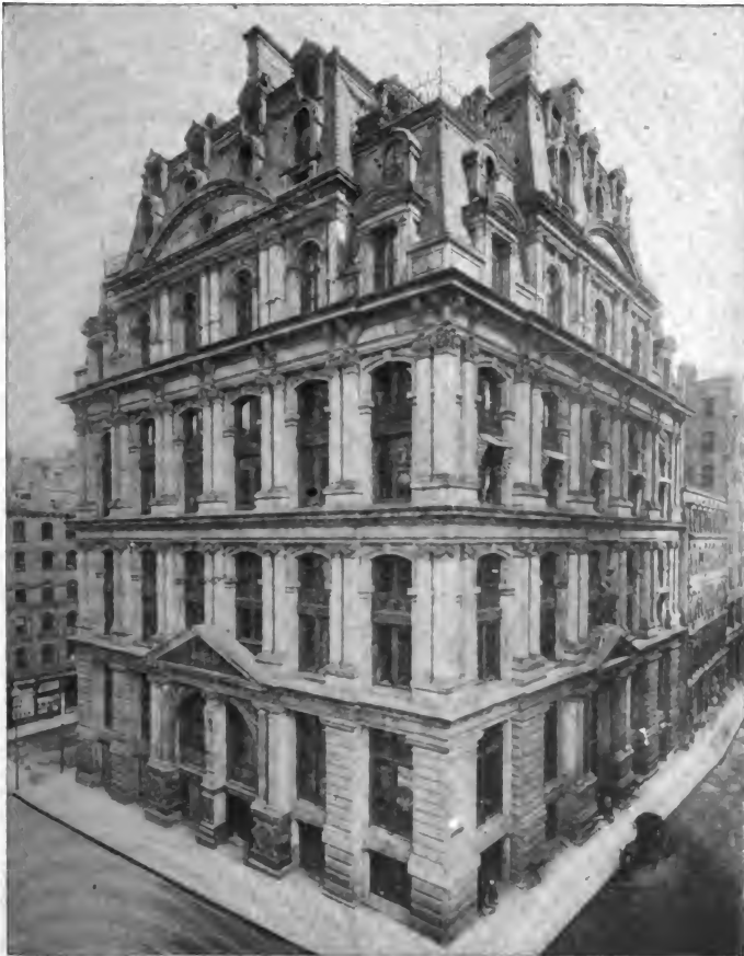
HOME OF THE NEW ENGLAND NATIONAL BANK, BOSTON.
